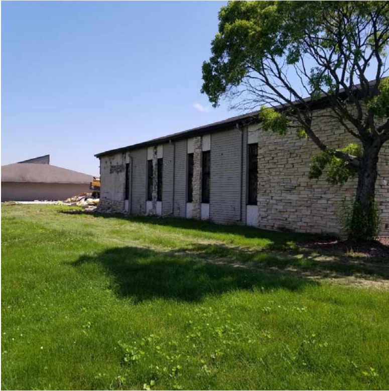
Image #6: West wall of the sanctuary
