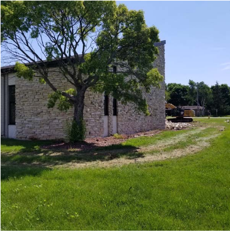
Image #5: South wall of the sanctuary viewed from the southwest.
