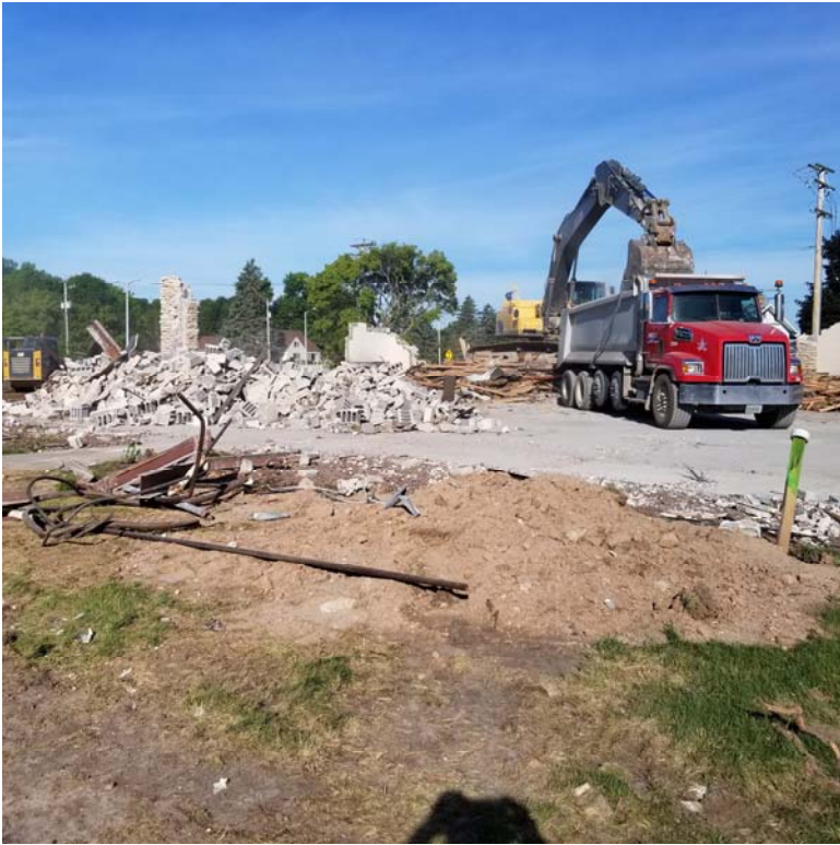
Image #10: Debris removal- looking from the northeast
