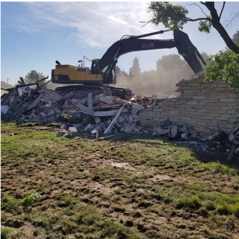
Image #4: Debris being removed at the southwest corner of the church..
