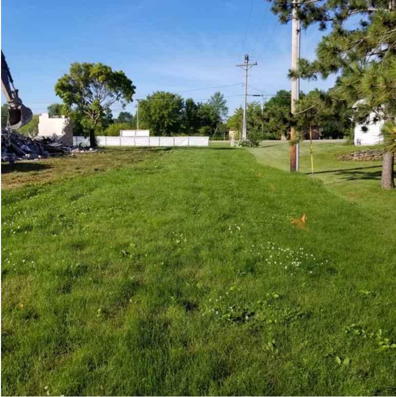
Image #5: West side of the site is being kept clean.
