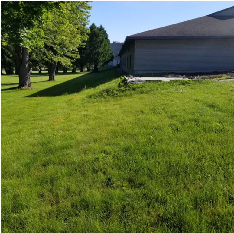
Image #6: West side of the site is being kept clean
