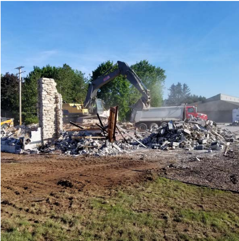
Image #8: Debris removal- looking from the southeast.
