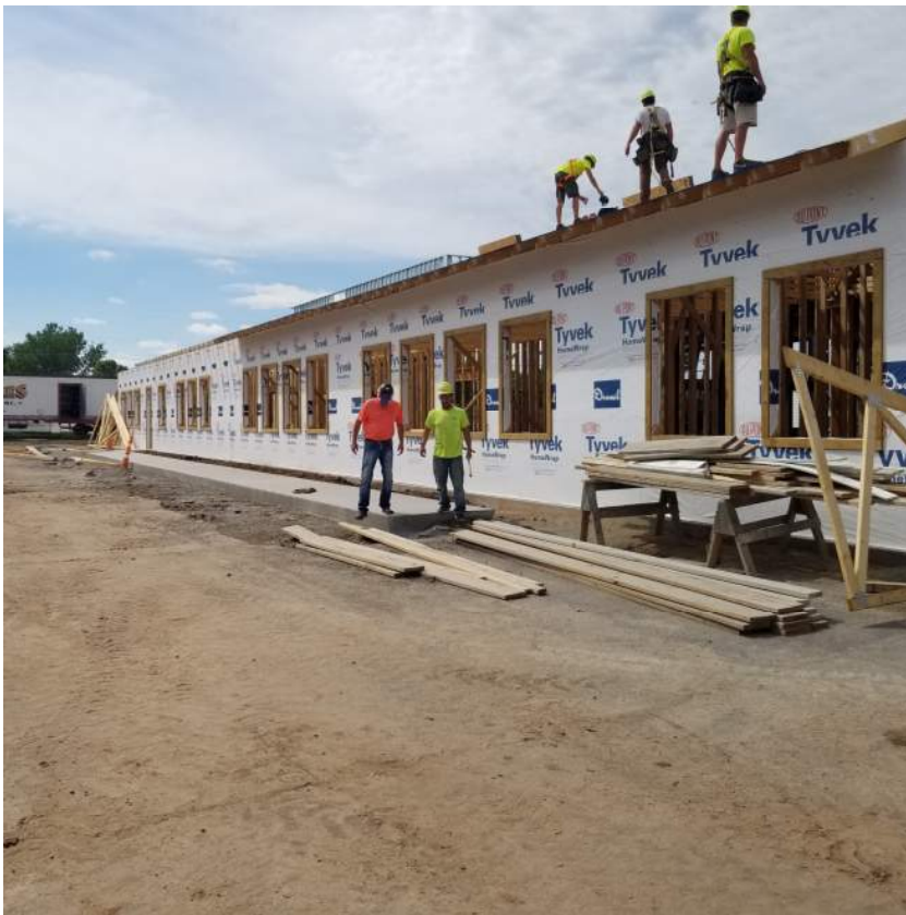
Image #3: Roof sheathing is being installed.
