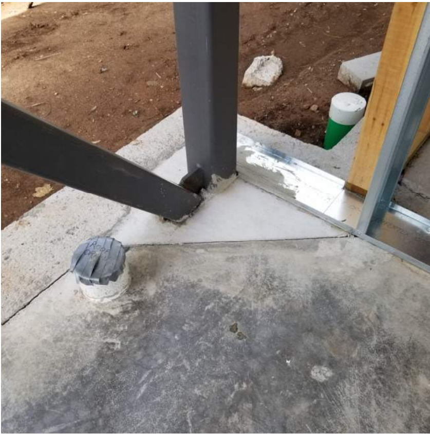
Image #7: Steel column bases have been grouted in place.
