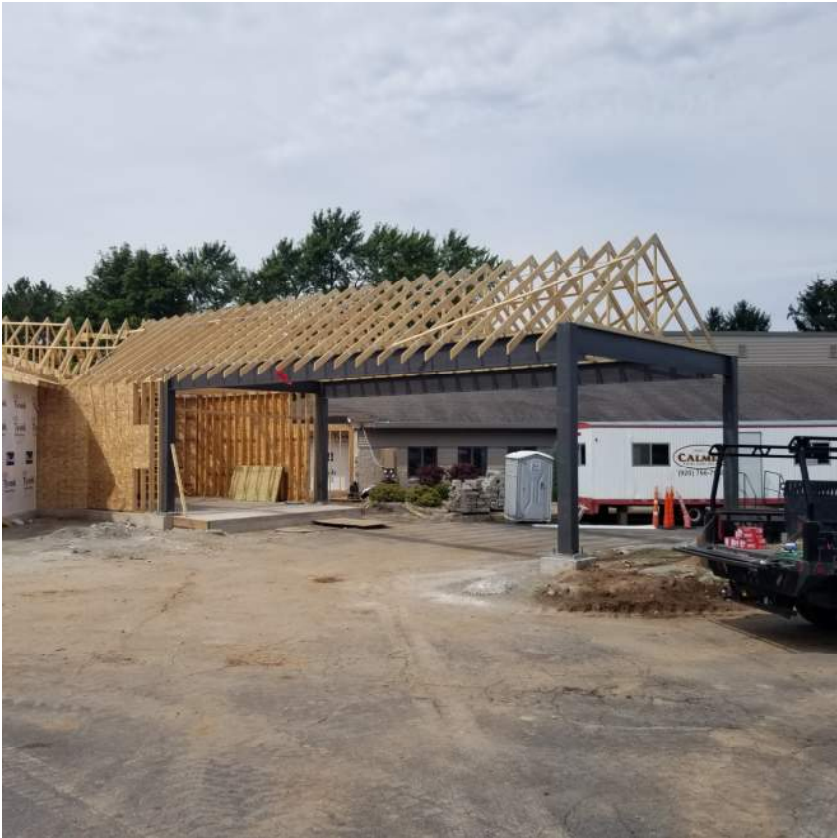
Image #2: Trusses have been set over covered drive area.
