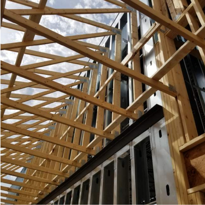
Image #9: Wood truss bearing on the east side of the church.
