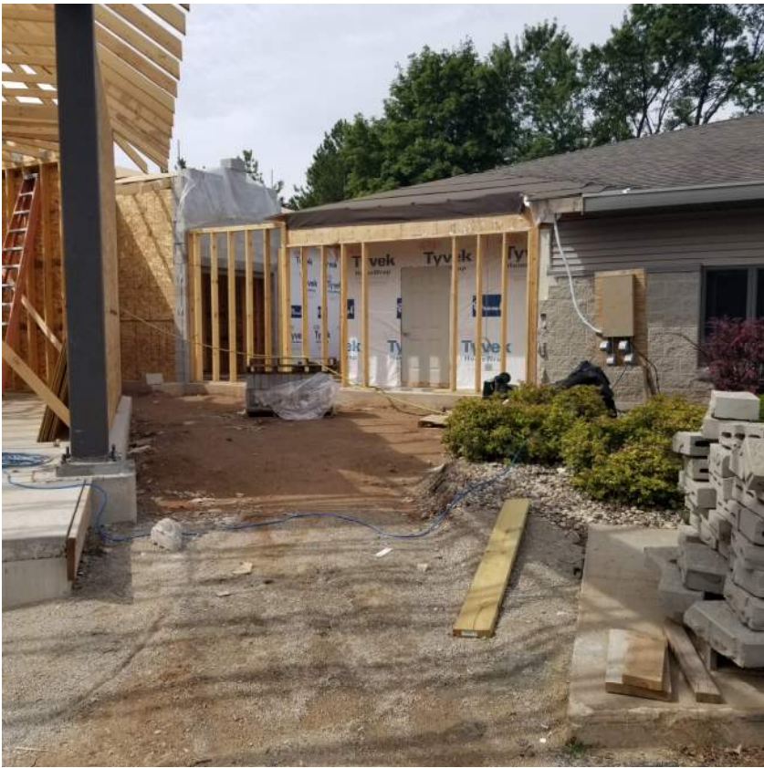
Image #1: Exterior wall @ previous building exit is now being framed in.
