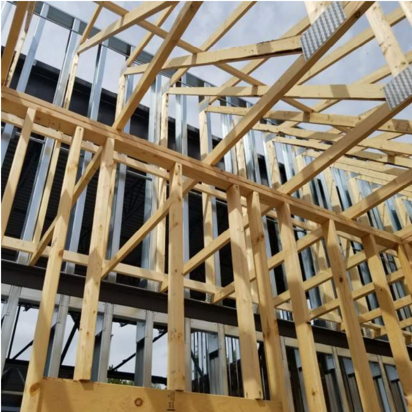
Image #10: Wood truss bearing on the east side of the church.
