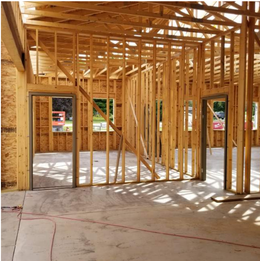
Image #4: Hollow metal frames are being set in place.
